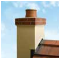
Brick or Stone Chimney (Class 1)
